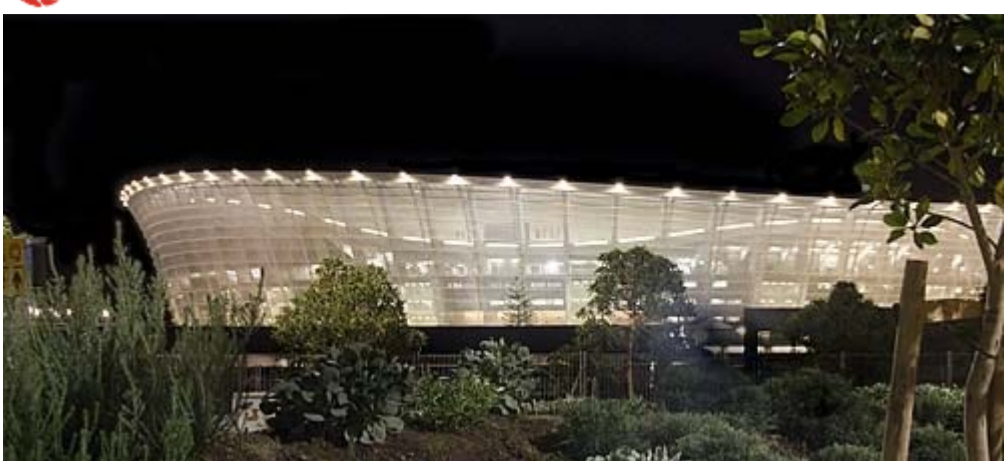
The Calm Before The Storm ~ Green Point Stadium just before kick-off
